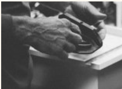
1947 - Torsten and Birgitta Mattson, representing the 4th generation of the family business, continue to search for ways to refine bed and mattress production, constantly looking for better filling materials and methods to improve the already high quality of their beds and mattresses.
